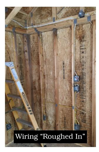
While I had other things I absolutely needed to do to be ready for the insulation (like install rafter vents and frame out the gable ends) Wednesday I started installing outlets, then switches on one of the two circuits. Finally, hoping to assuage my growing doubt, I stood in front of the panel, put my finger on the breaker then flicked the switch and...*nothing* happened. Which is good, which is what you want. Then,
