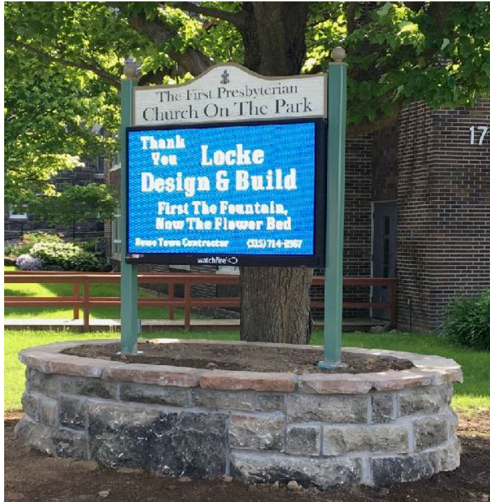
Recently completed “Flower Fountain” around the new sign, built by Tyler Locke, grandson of Gene and Shirley Seeley. Flowers will be planted soon.
